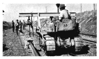
Crawler tractor, with rail threader suspended from beam, lifts rail to centre of track.
