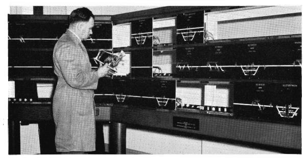
All Centralized Traffic Control equipment has arrived from England and is being assembled by the contractor, McKenzie & Holland (Aust.) Pty. Ltd. Fitter is shown installing a panel in the Australian-made illuminated track diagram in the Traffic Control room at Head Office.
