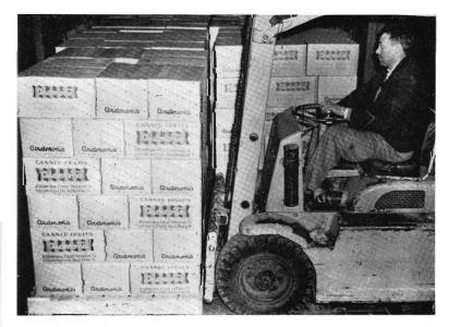
THEY'RE STUCK! Foods in cartons—such as tinned fruit and condensed milk—are now being carried in pallet size loads, as shown above. The cartons are held together by a special adhesive, in such a way that they are resistant to train movements but can easily be separated on arrival at destination. Each pallet load of tinned fruit weighs just over 1½ tons. This method eliminates the steel strapping of cartons at factory and also facilitates handling of goods in transit.
