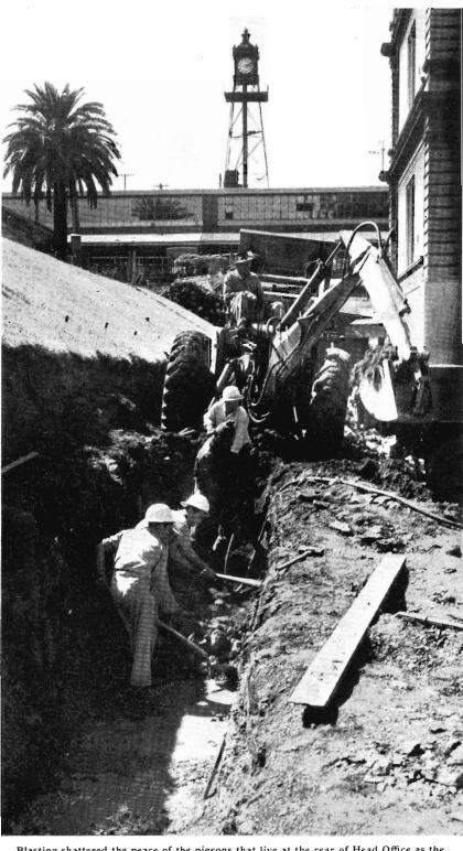
Blasting shattered the peace of the pigeons that live at the rear of Head Office as the channel and tunnel for this drain were cut. The drain, 1.516 ft. long and up to 20 ft. deep in parts will provide drainage for the new Spencer Street station and subway. It was necessary to cut 200 ft. of tunnelling, part of it through the embankment at the rear of the offices.
