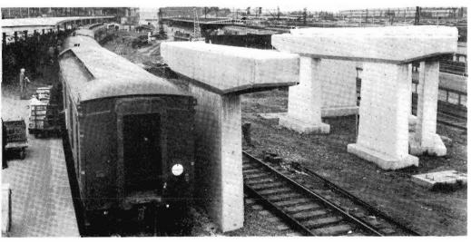
Concrete piers and cross-heads for the vehicular overpass leading from the inner car park to Spencer St.
