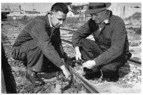
TESTING: Electrical Fitter-in-Charge J. D. Morelli (left) and assistant R. McLure, of Traralgon, check the insulating block joint between adjoining track circuits. This is done by connecting rail joints in a circuit with dry cell; any leakage is revealed by deflection of a voltmeter needle.
