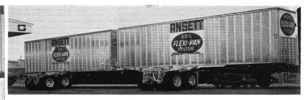
(Above) Double Flexi-Van: The first double Flexi-Van goes into service. The wagon, 75-ft. long, carries two 35-ft. Flexi-Vans and is the first of ten to be used by two of Australia's major transport operators on the standard gauge line.
